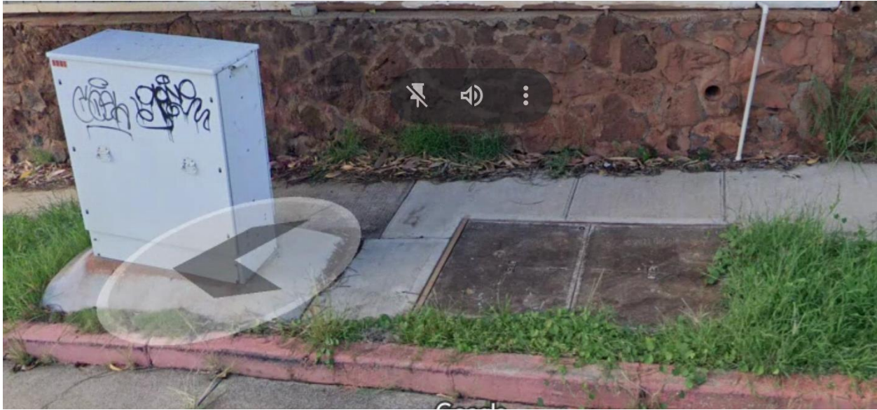
Figure 5: Example of a location where underground broadband is surfaced to a conduit to serve a household
